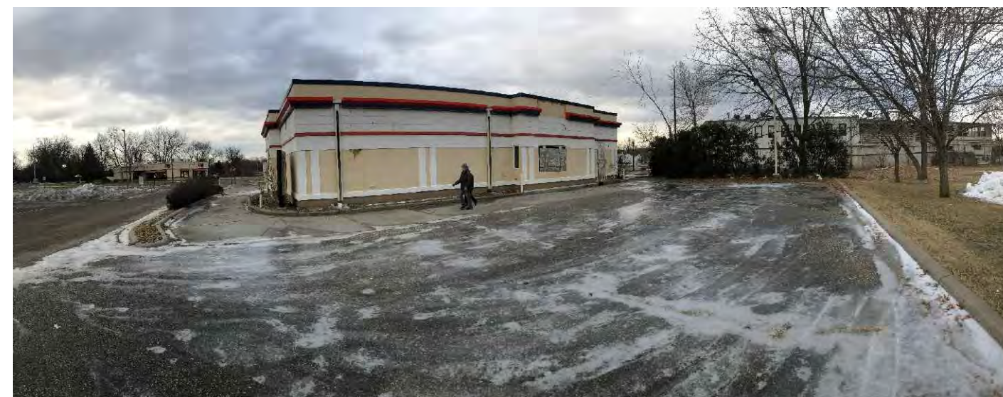
EXISTING CONDITIONS PHOTOS
