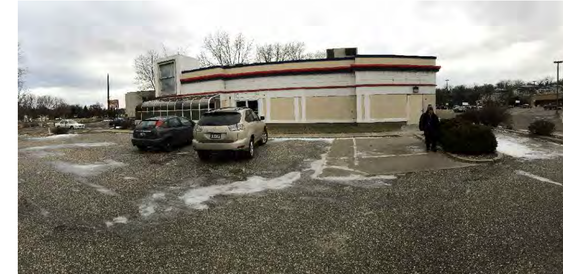
EXISTING CONDITIONS PHOTOS
