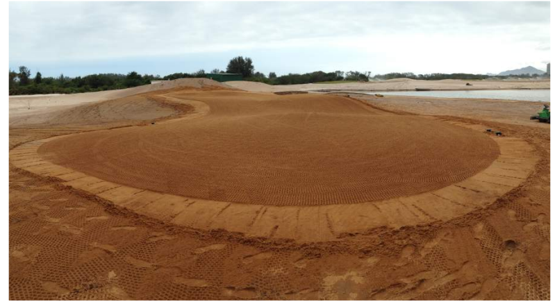
Finishing a green built out of pure sand green at the Rio Olympic Golf Course. The process will be a little slower in Chaska!
