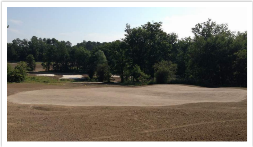
Finishing a heavily undulating green in the heavy wine country soils of St. Emilion, France. Shaping by Renaissance Golf Design Associate Brian Schneider.
