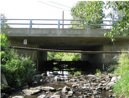
East Side View – Bridge L2724
