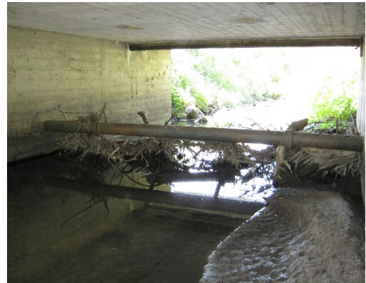
Sanitary Pipe Suspended Beneath Bridge Deck
