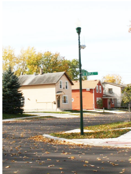
New Fiberglass Street Lighting
