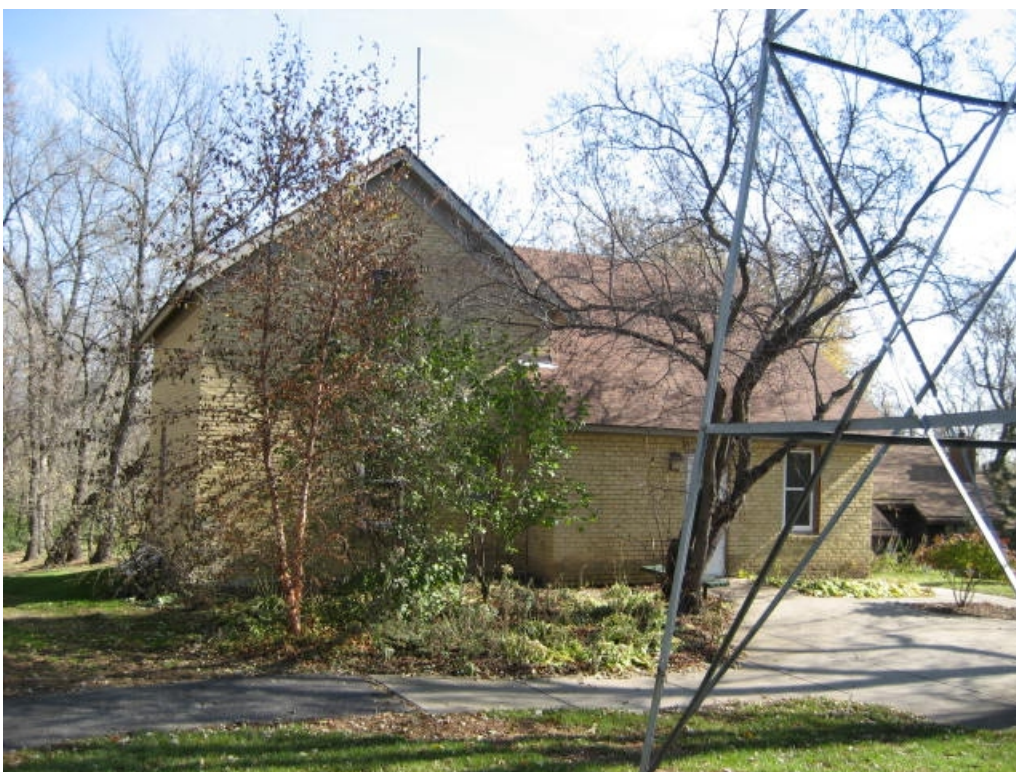
Front Elevation of the Eitel House
