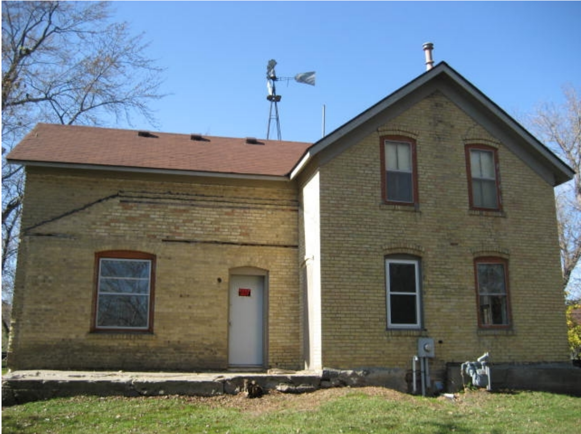
Rear Elevation of the Eitel House
