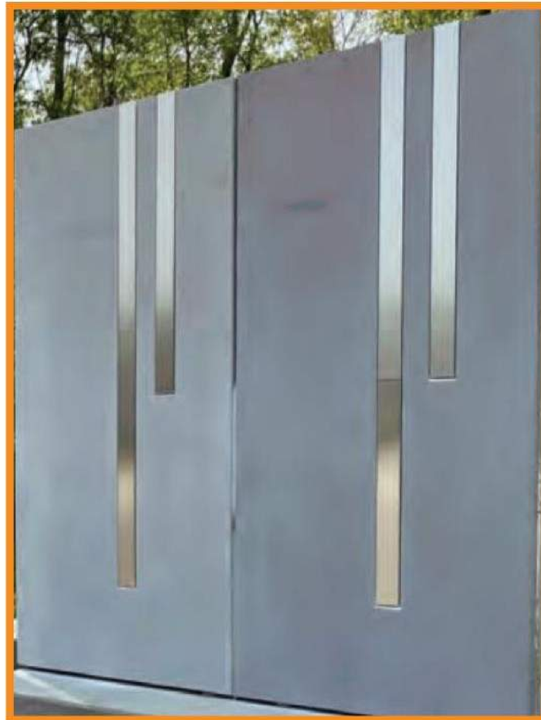
Stainless steel elements inset into the precast panel reveals.
