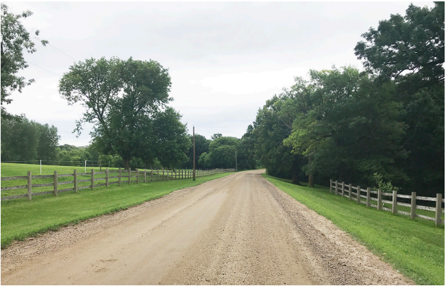
PHOTO: EXISTING CONDITIONS MARSH LAKE ROAD (RURAL)
