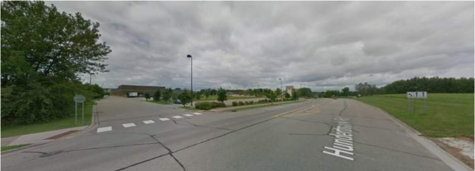
EXISTING VIEW - HUNDERTMARK RD SOUTH
