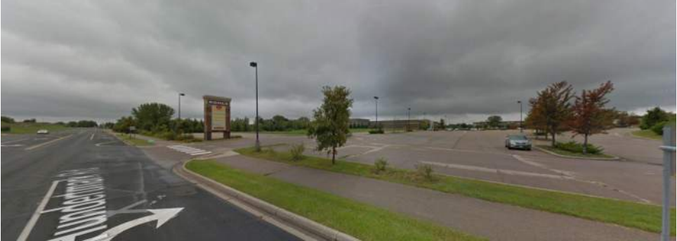
EXISTING VIEW - HUNDERTMARK RD EAST ENTRANCE
