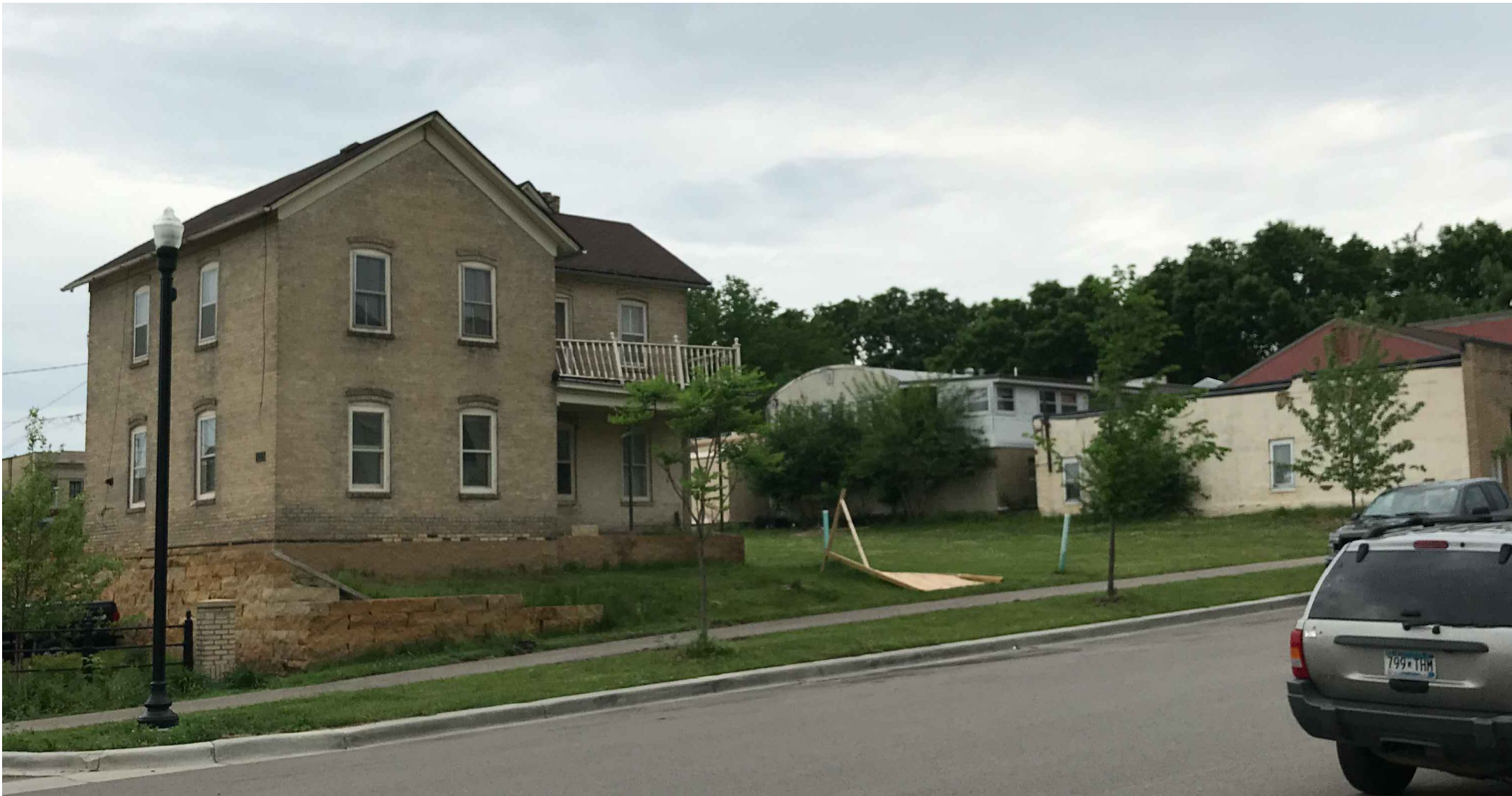
1 SITE VIEW FROM SOUTHEAST A800 N.T.S.
