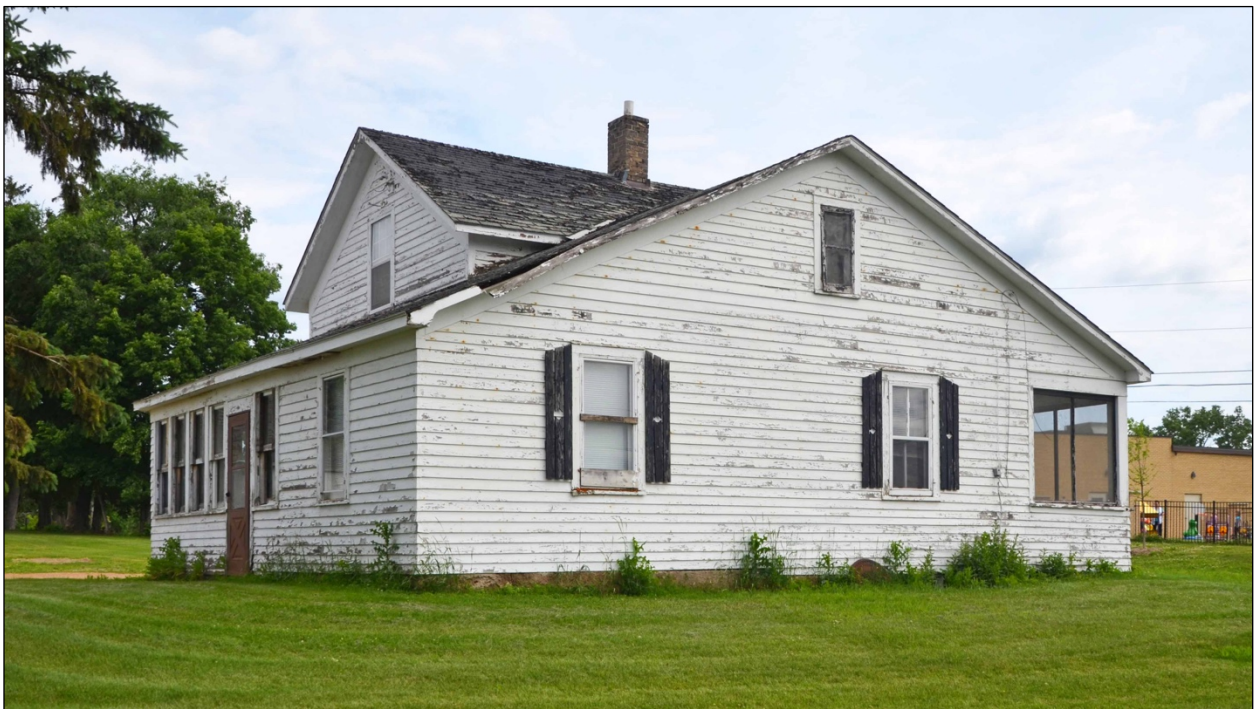
Photo 14. West and south elevations.
