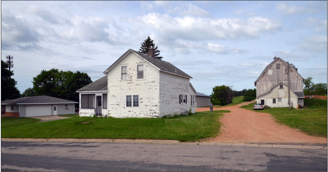
Photo 7. Overview of the site, looking southwest.
