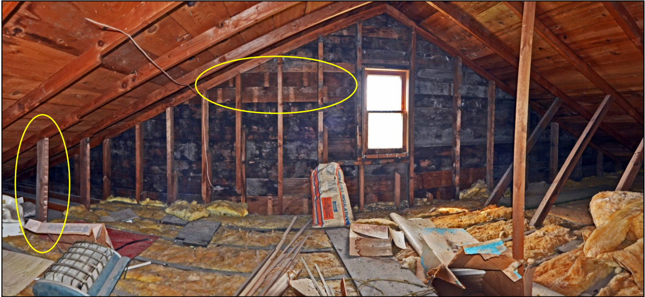
Photo 17. Attic of the porch wing, looking south. Note stud and lath “shadows” on sheathing boards and studs, indicating that the lumber has been recycled.
