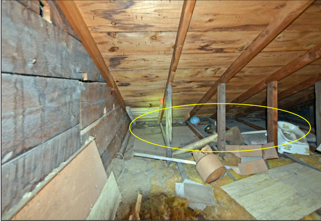
Photo 19. Attic above the porch wing, looking east. The wall of the original house is visible at left. Note new framing and sheathing over the front porch.
