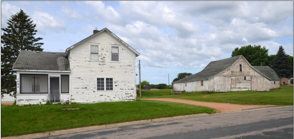
Photo 8. Overview of the site, looking west.
