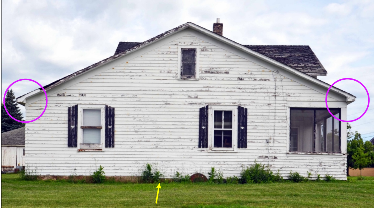
Photo 15. South elevation. Compare roofline to the original, shown in Photo 9. Soffit details at intersection of eaves and rakes are typical of post-WWII construction. Jog in the siding (arrow) marks change in the foundation. Original foundation is to the right, slab-on-grade foundation to left of arrow was built to support the addition.
