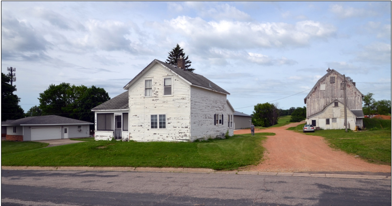
Photo 7. Overview of the site, looking southwest.
