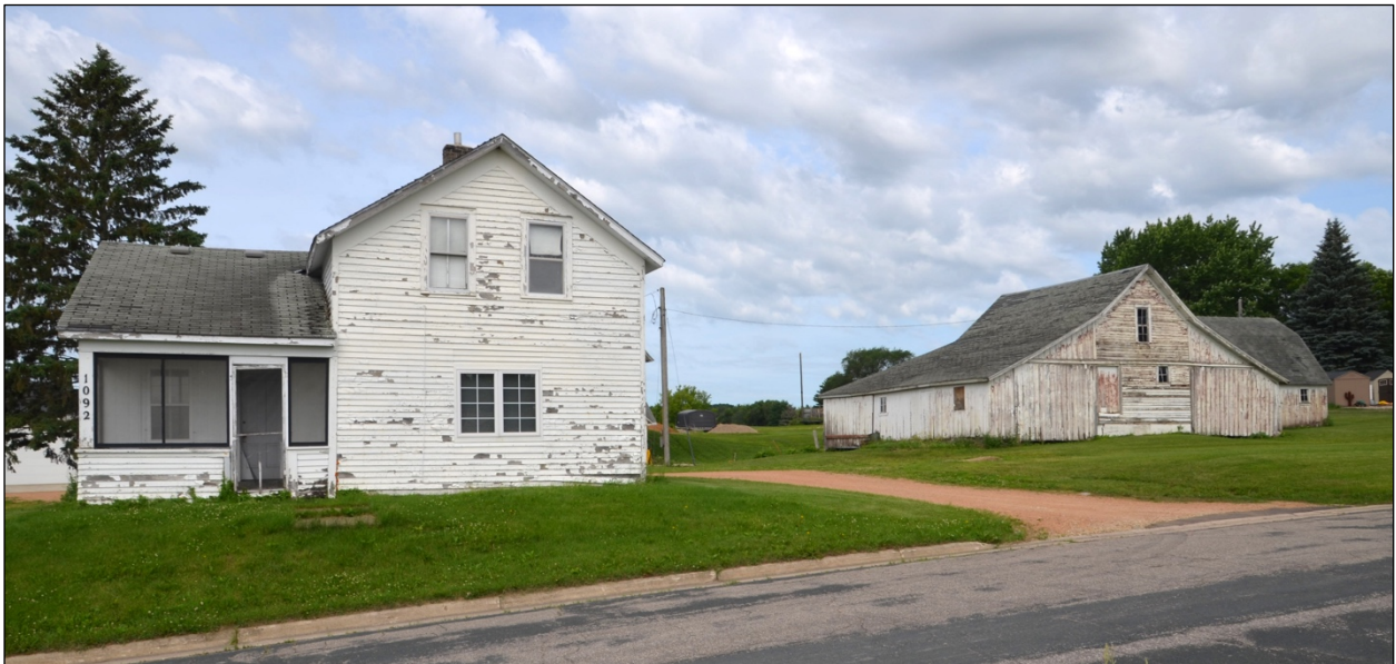
Photo 8. Overview of the site, looking west.
