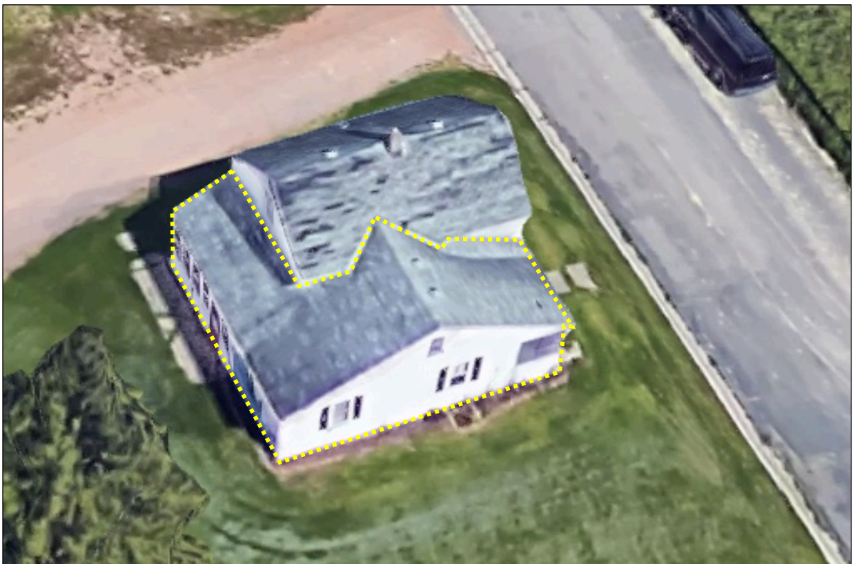
Photo 6. Birdseye view, showing west and south elevations. Addition is outlined.
