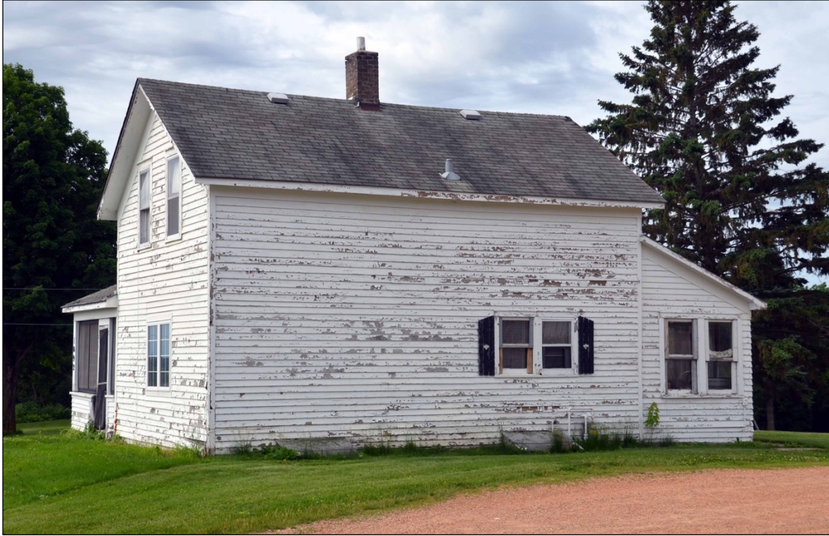
Photo 11. Principal (east) façade and north elevation.
