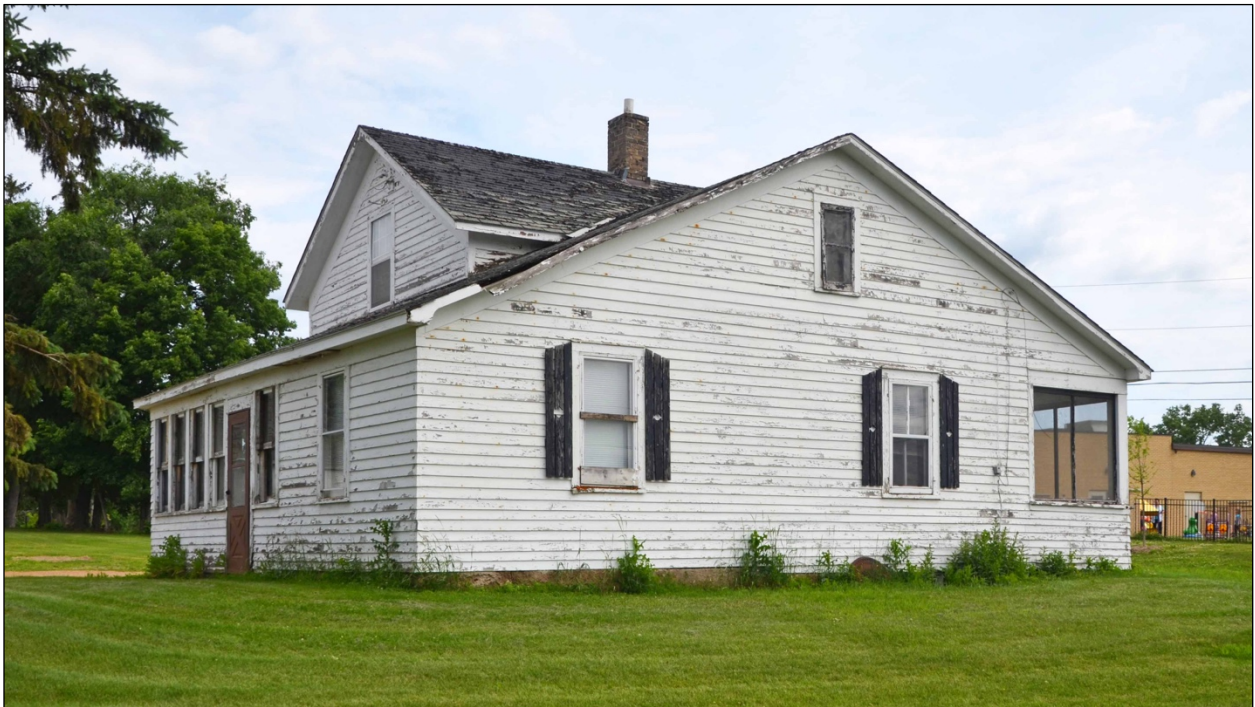
Photo 14. West and south elevations.
