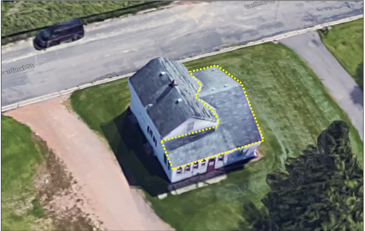
Photo 5. Birdseye view, showing north and west elevations. Addition is outlined.
