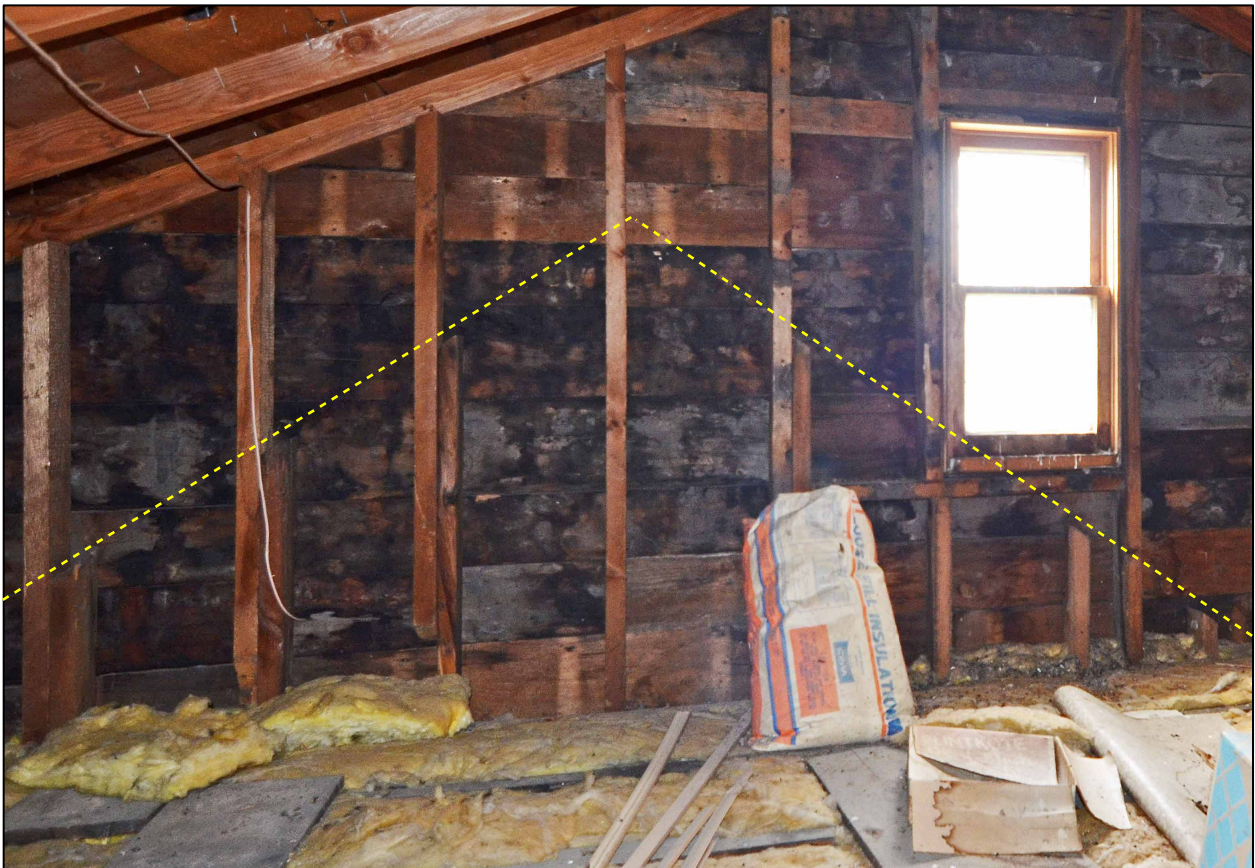
Photo 18. Close up of attic above the porch wing. Original studs remain in place, showing roofline of original porch wing. New studs were scabbed onto the originals when the wing was expanded.
