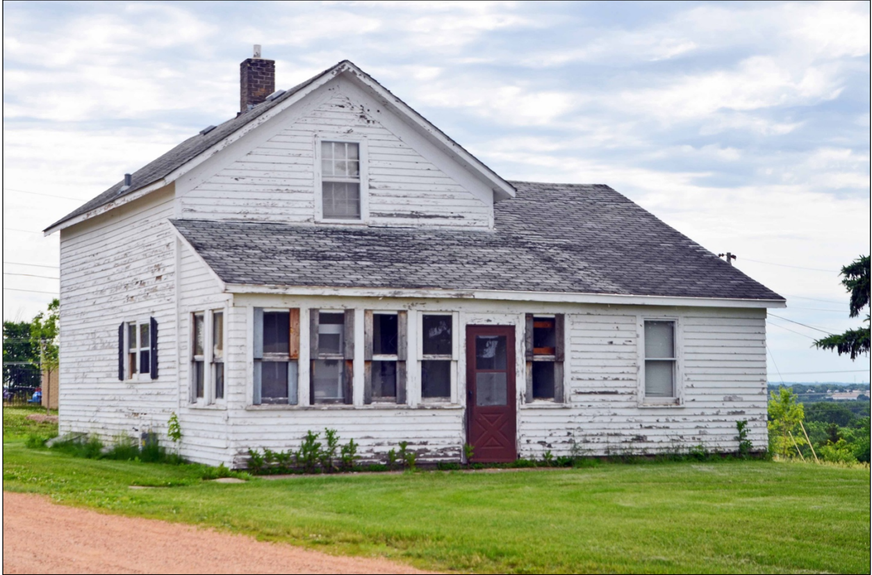
Photo 13. North and west elevations. Double-hung 6/6 sash on upper level may be original.
