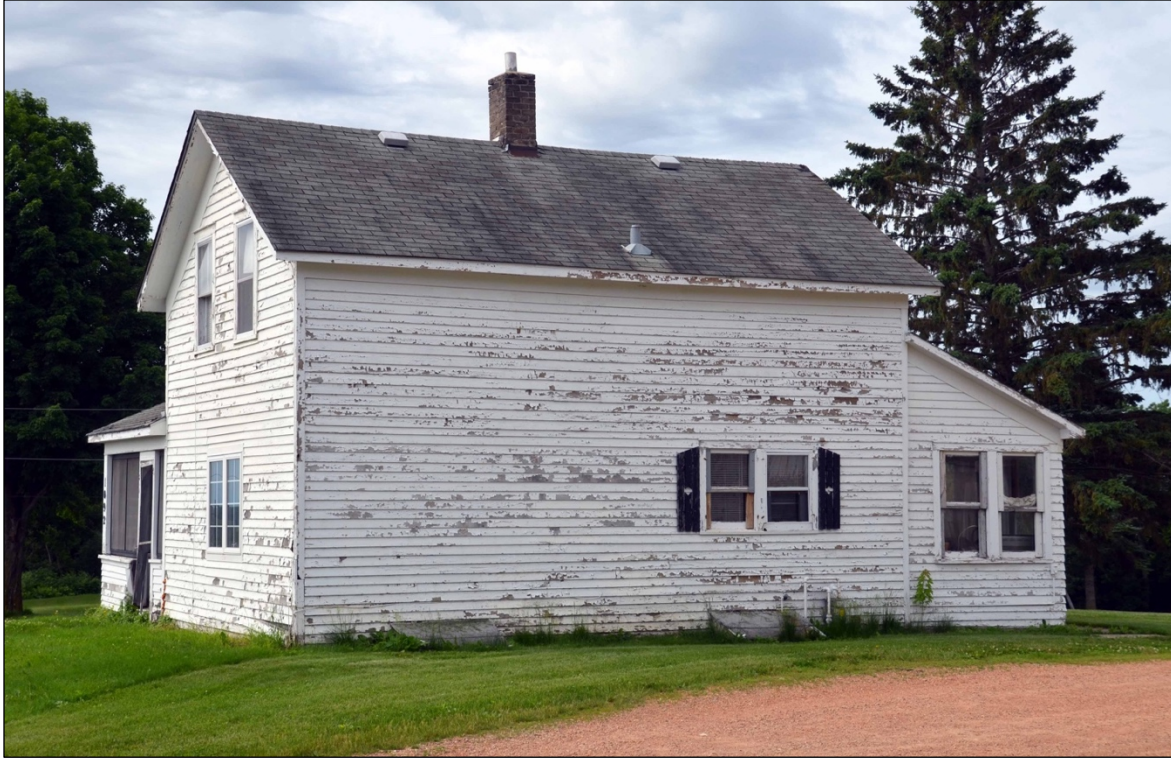
Photo 11. Principal (east) façade and north elevation.
