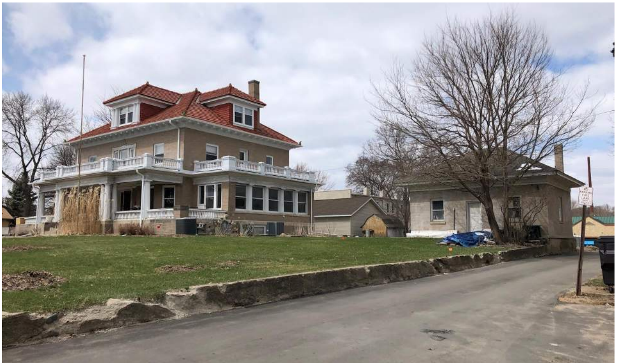
View from 4 th at alley
