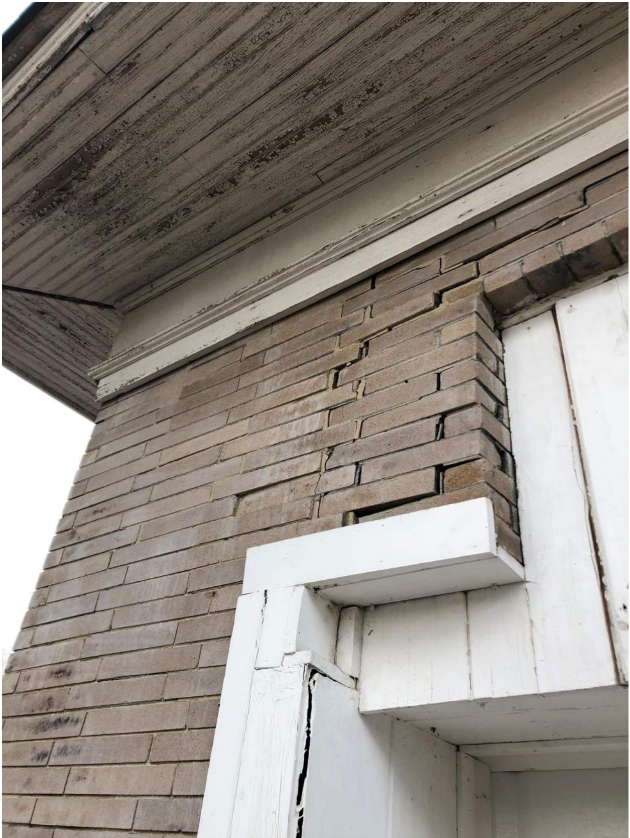
Close-up of northwest corner
