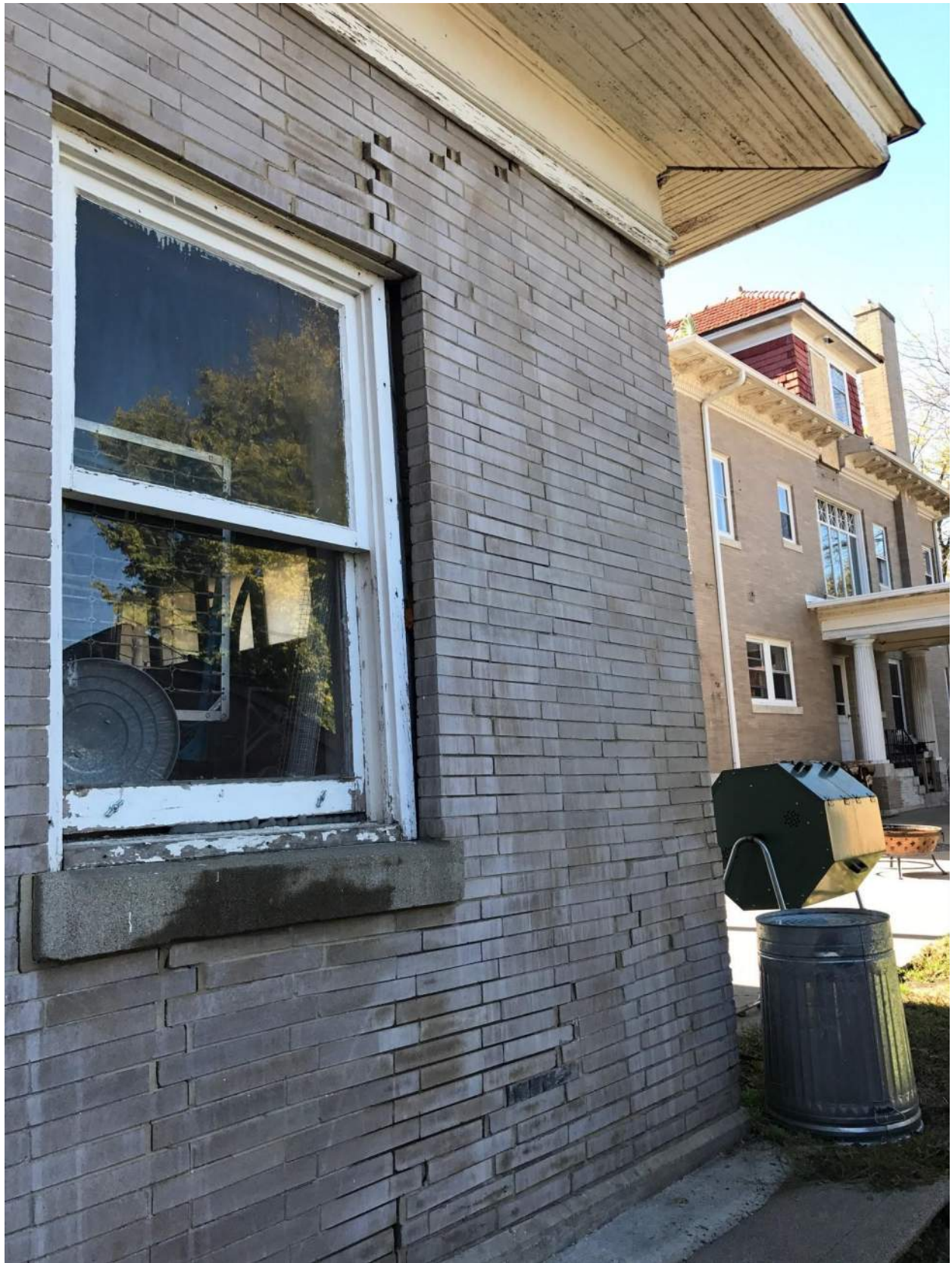
View of northwest corner
