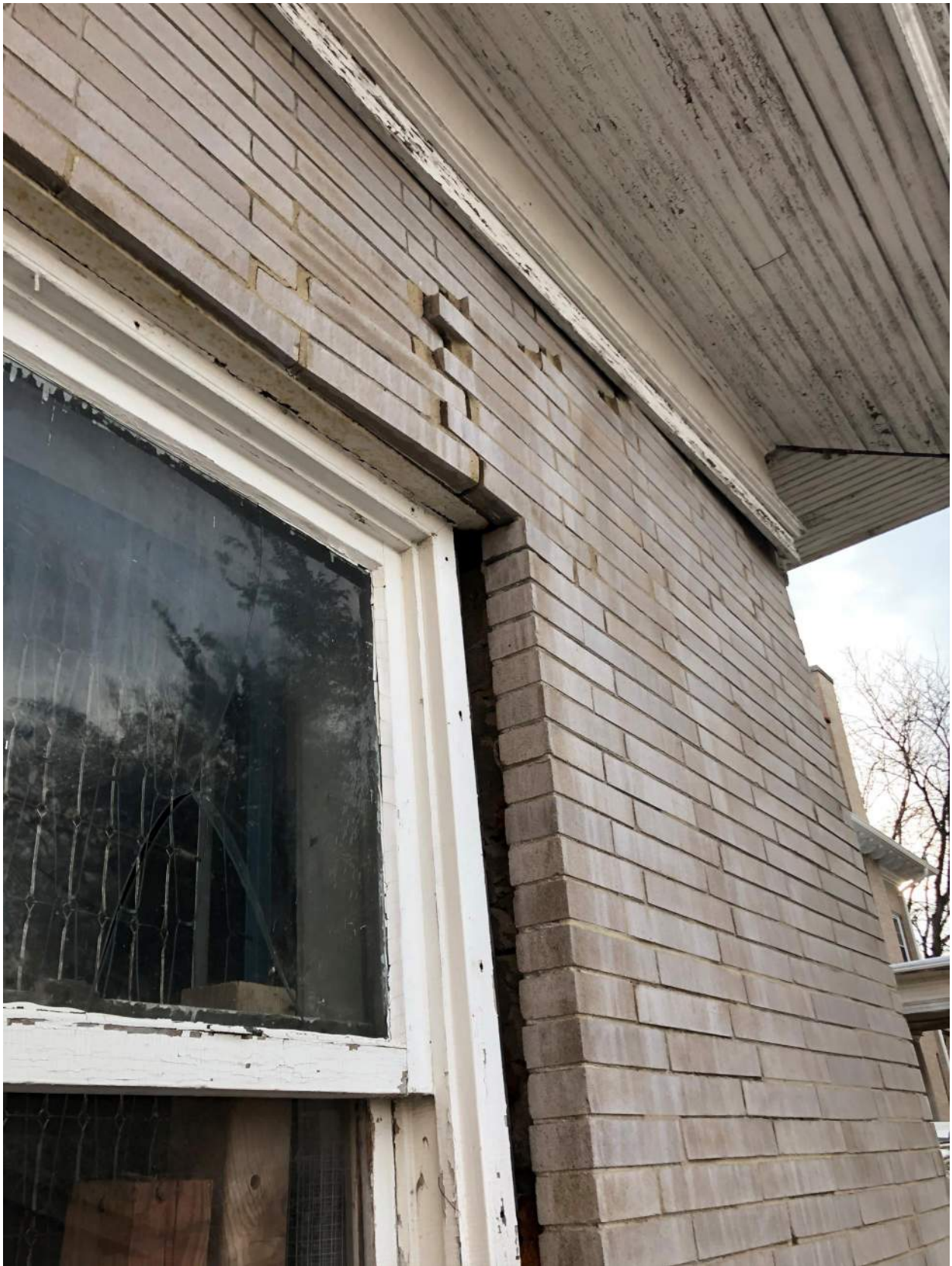
Close-up of northwest corner
