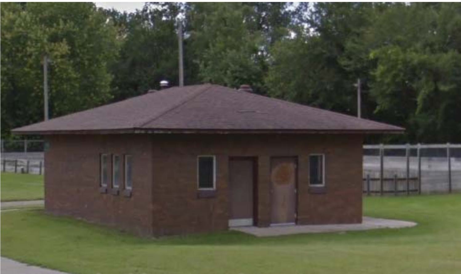
Existing building - north entry
