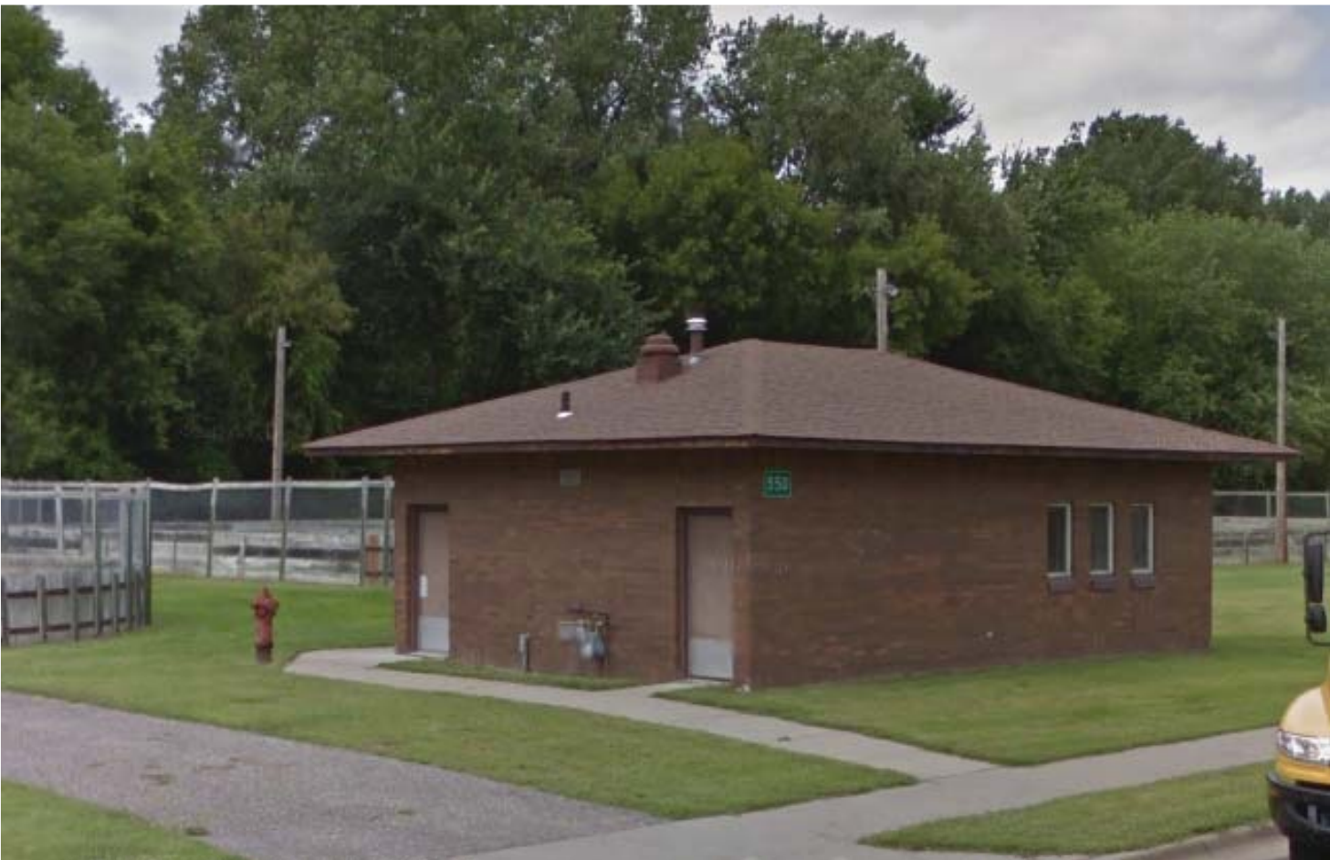
Existing building - south elevation
