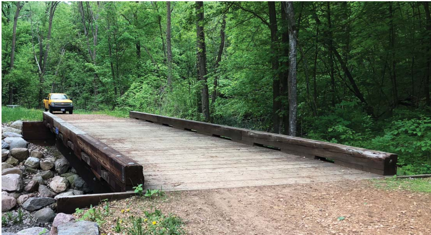
Example of Chaska trail bridge
