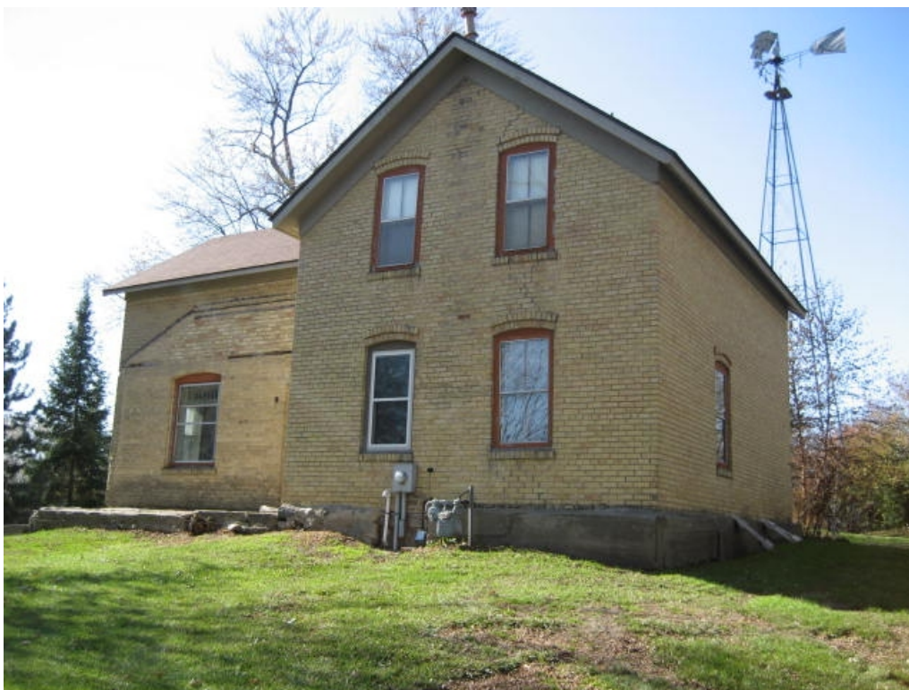
Rear Elevation of the Eitel House
