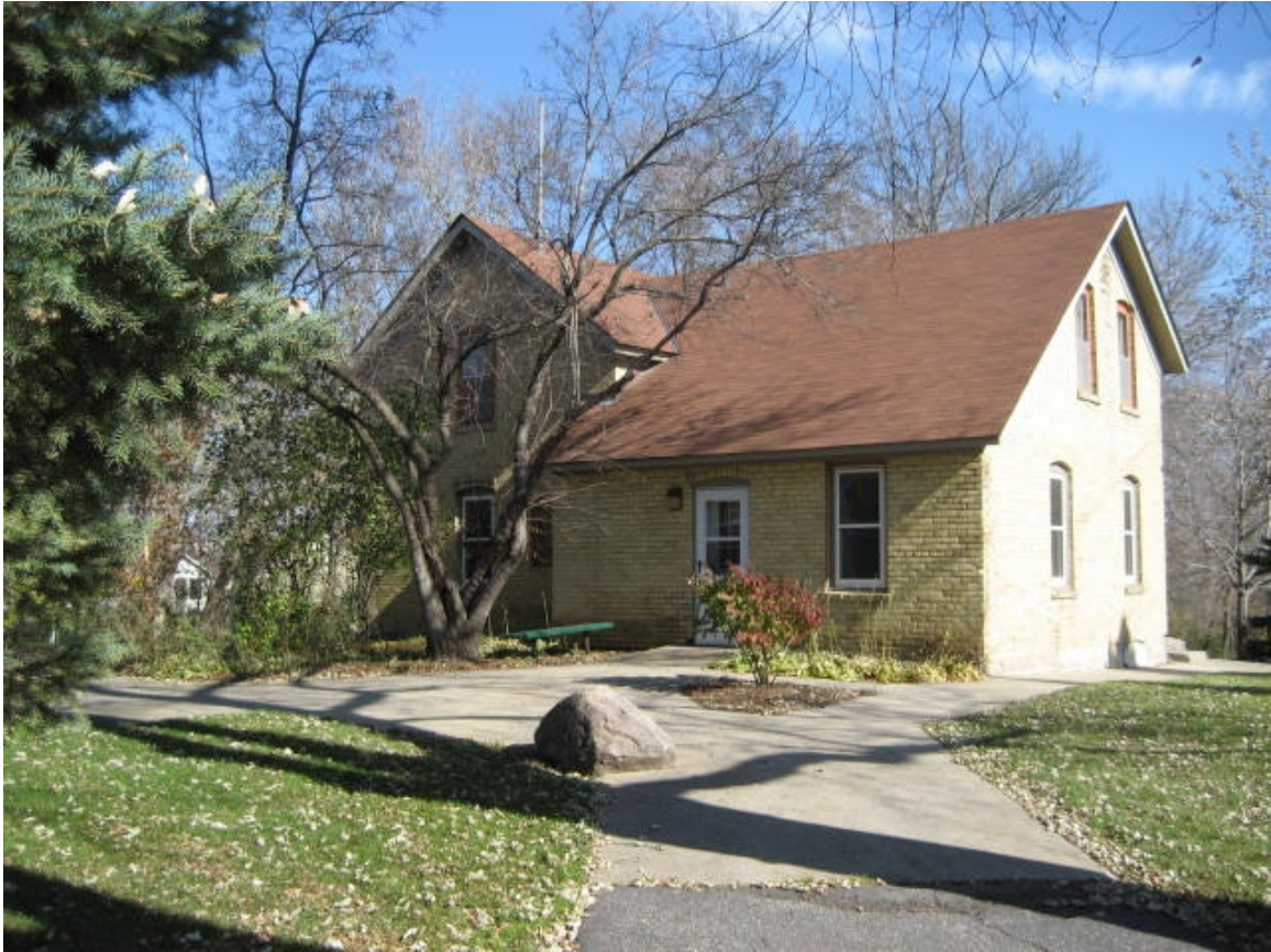
Front Elevation of the Eitel House
