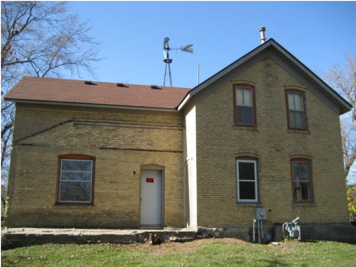
Rear Elevation of the Eitel House
