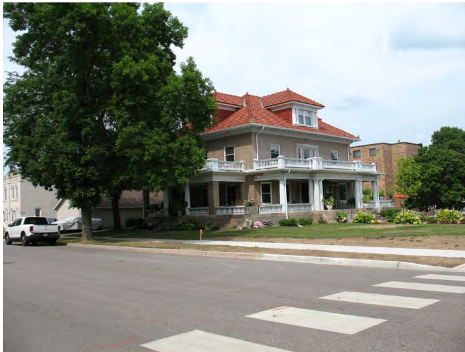
Christian P. Klein House, 205 East 4 th Street, view to northeast. Although materials have been replaced, the street, curbs, and sidewalks along Walnut Street retain their historic configuration.
