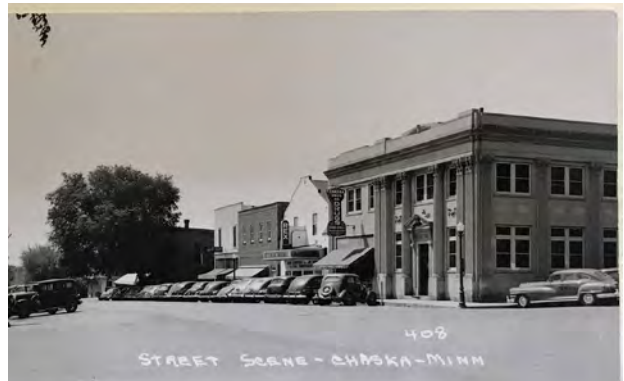
First National Bank, 213 Chestnut Street, 1940. View to southwest.
