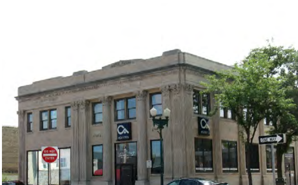
First National Bank, 213 Chestnut Street. View to southwest.
