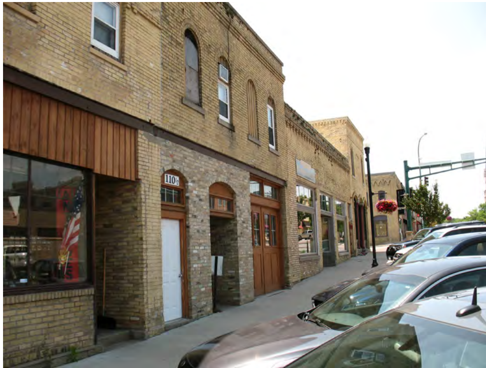
Commercial buildings along East 2 nd Street, view to southwest
