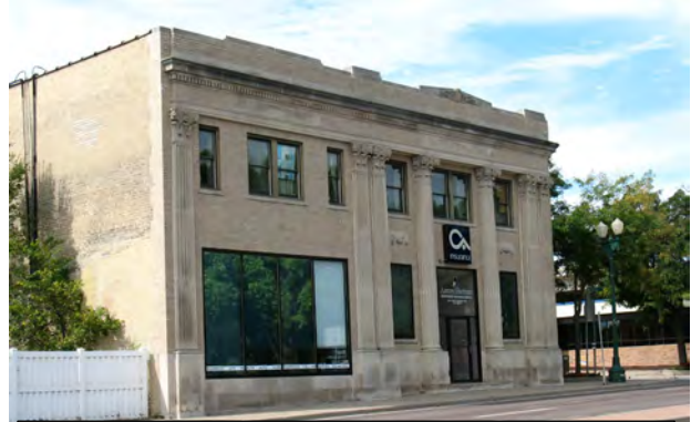
First National Bank, 213 Chestnut Street. View to northwest.
