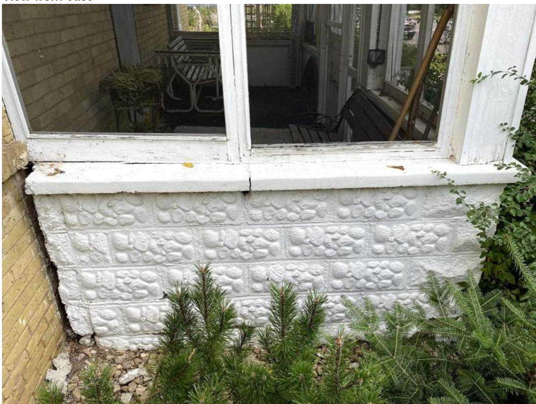
Porch pulling away from house due to deteriorating foundations
