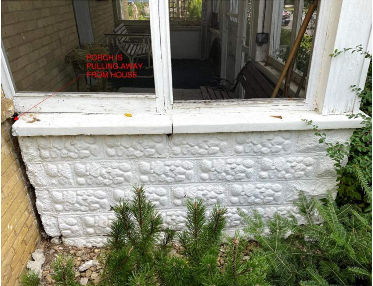
Photo of the west face of the existing porch. Note the "cobblestone" faced concrete blocks.
