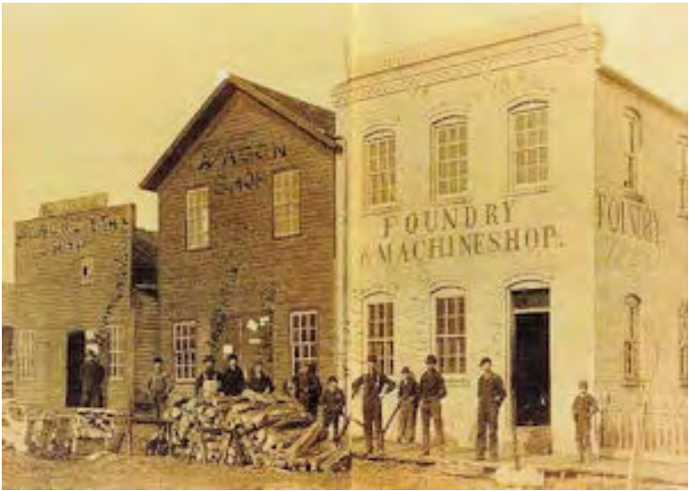
Ess Bros. Foundry
