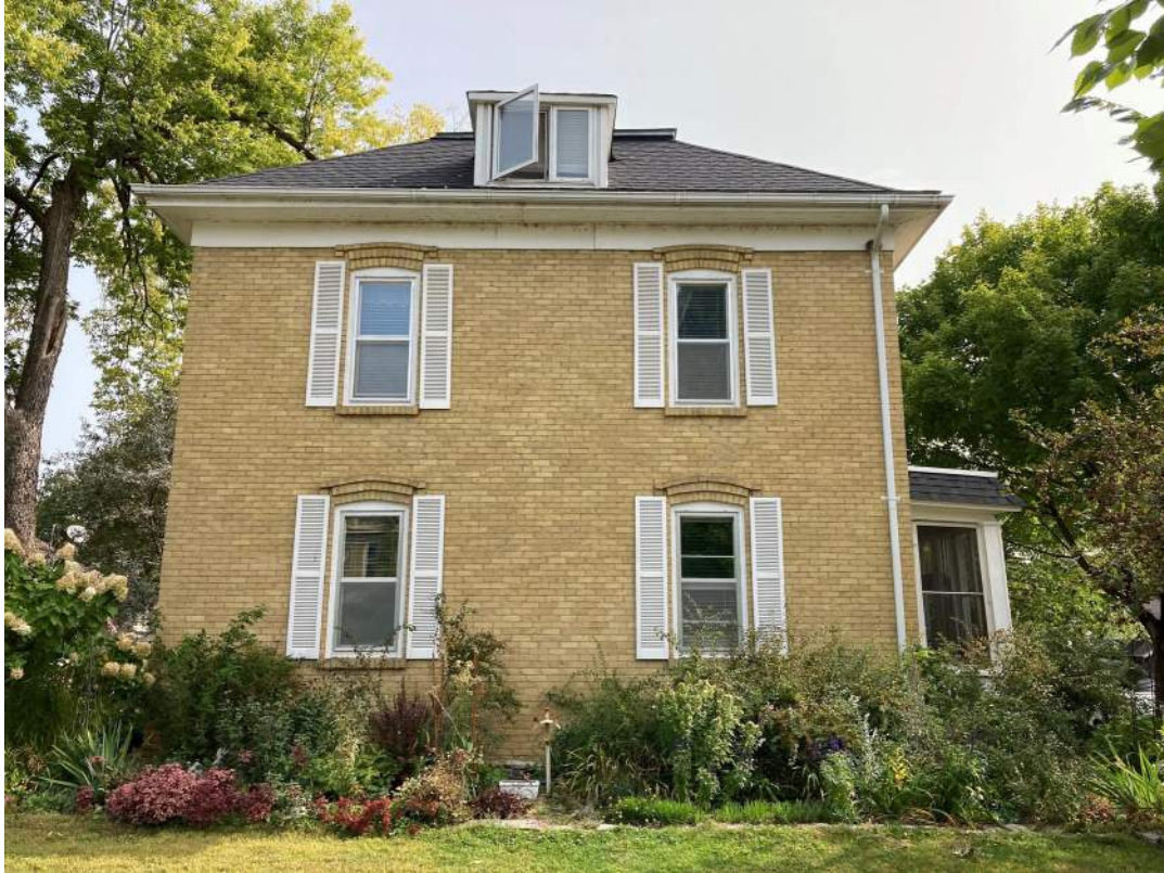
View from west (Elm Street)
