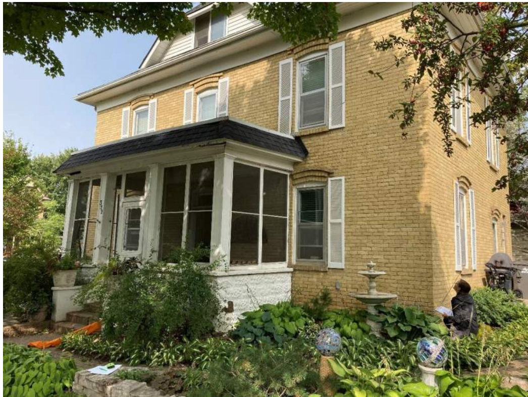
Existing porch is situated tightly between flanking first floor windows
