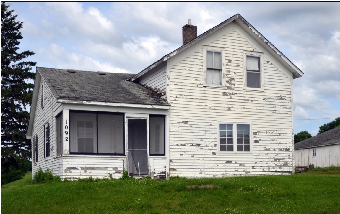
Photo 10. Principal (east) façade and south elevation, 2018. Note the changes to the porch as well as window and door openings. Original 6/6 sash have been replaced by 2/2 and 1/1 on upper level and modern crank-out windows on lower level. Chimney above the porch wing is gone and chimney above main section of the house has been altered.
