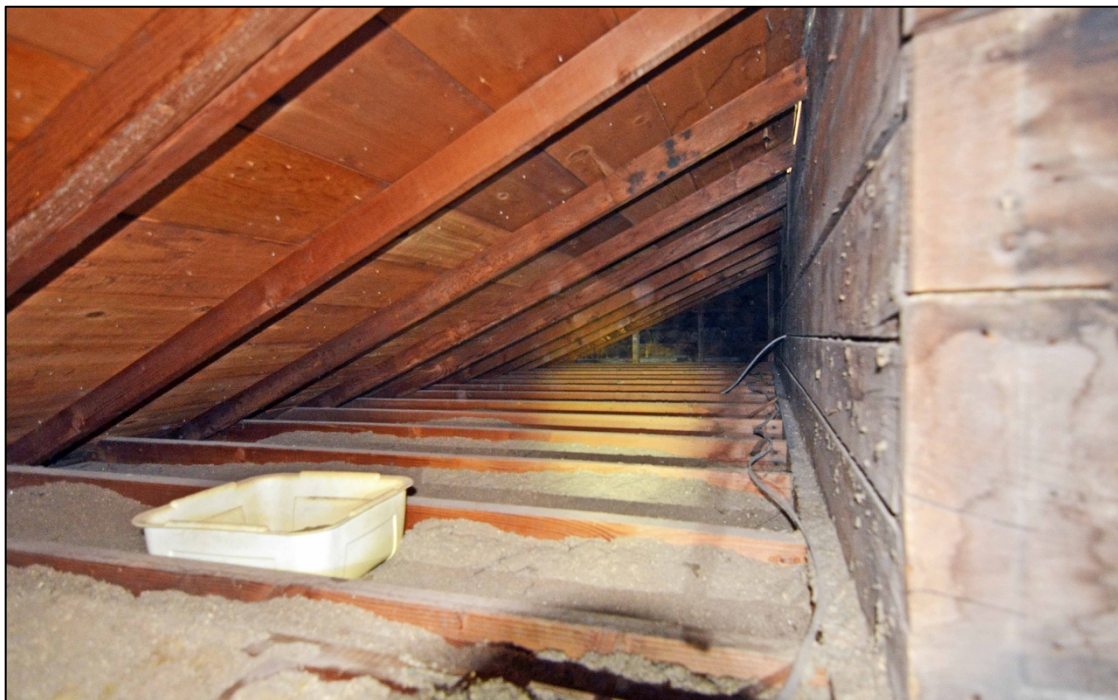
Photo 20. Roof framing above the west bay of the addition. Wall of the original house is visible at right. Roof framing here and elsewhere in the addition is smooth-surfaced, nominal 2 x 4 lumber typical of the mid-twentieth century rather than rough-sawn, full dimension lumber that would have been available at the time of the home's original construction.
