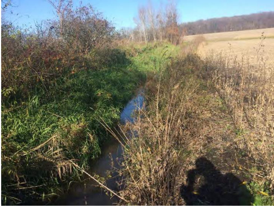
Channel 1 (photo facing north)
