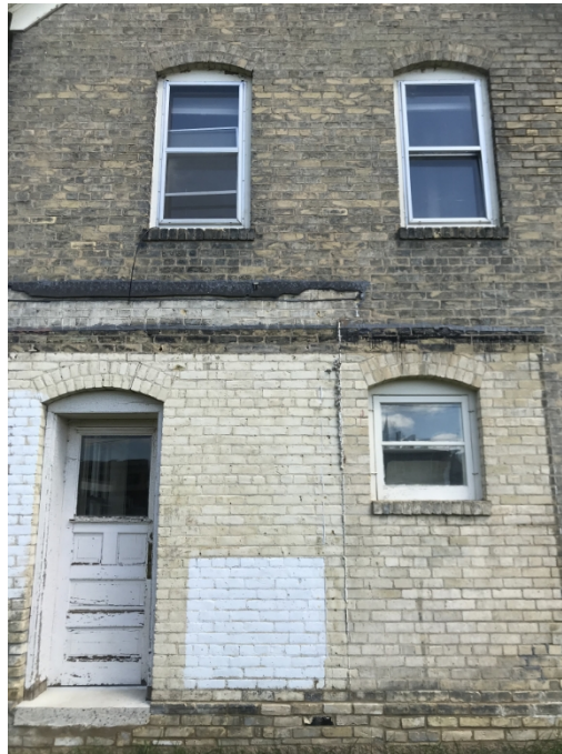
(Rear façade showing roof flashing of a potential previous addition)
