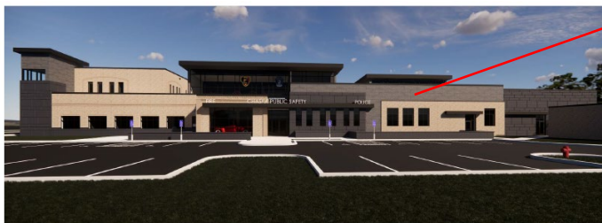
Figure 4: West elevation - Police Station
