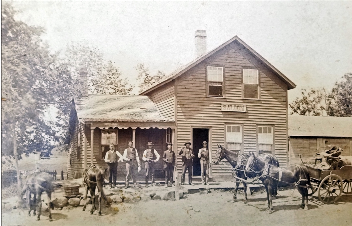
Photo 9. Undated early historic view of the house, when it served as a saloon. Note the wide skirtboard at the base of the wall.
