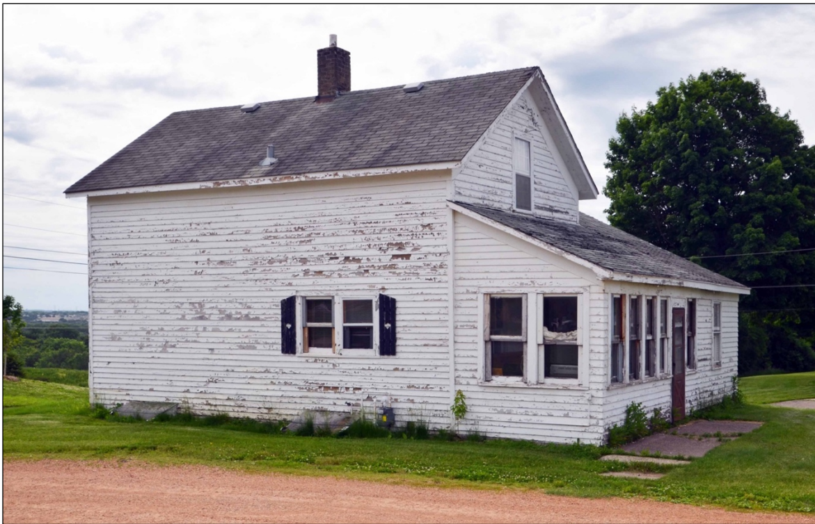
Photo 12. North and west elevations. The one-story bay at right is an addition. Clapboards of original house terminate at corner boards. Clapboards at corner of addition have metal corners. Clapboards on the addition do not align with clapboards on original house.
