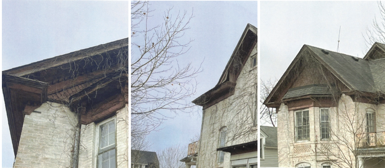
(images showing soffit/fascia and windows)
