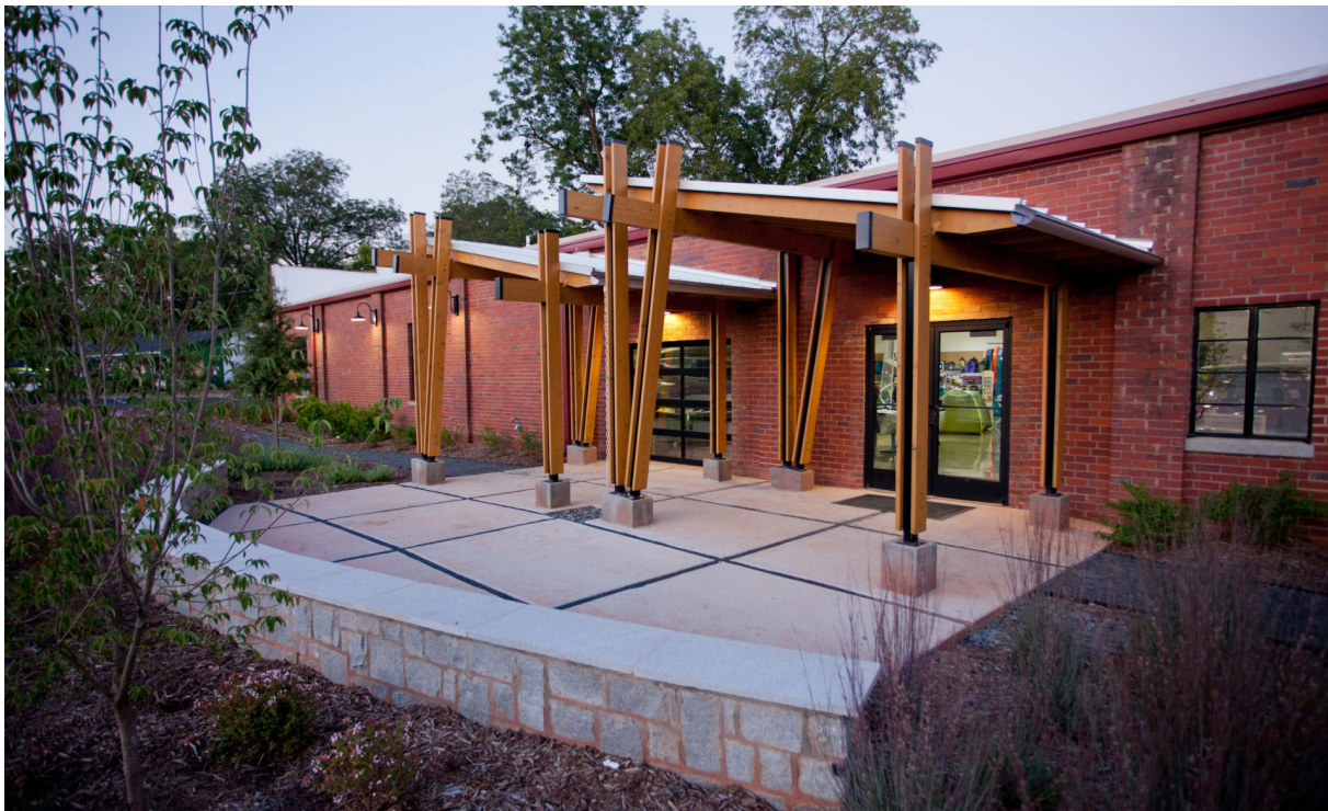
The side facade of this commercial building was retrofitted with an attractive trellis structure to call attention to the business entrance. An outdoor patio and landscaping was also integrated into the design. (Photos: Arcollab)
