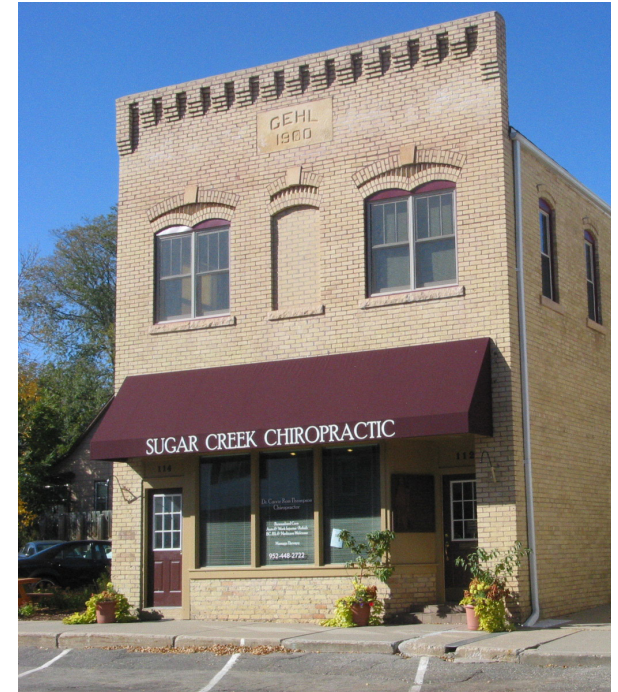
Recommended example of an awning with integrated business sign from the Downtown Chaska Signage Design Guidelines.
