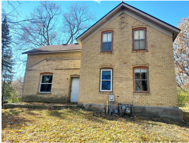
(Rear elevation of home showing previous porch markings)
