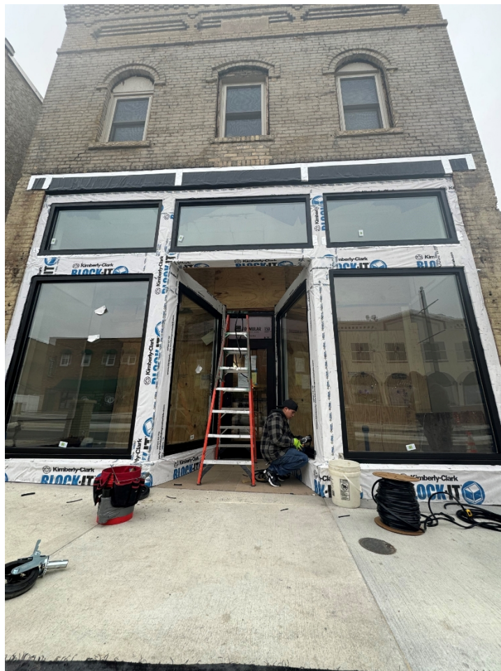
(Image taken January 2024; storefront improvements)
