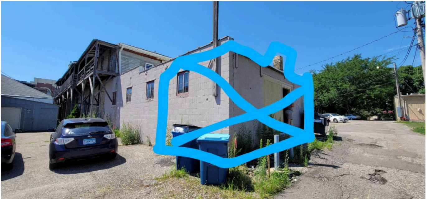
Rear view showing the portion of the building being converted to an outdoor patio
