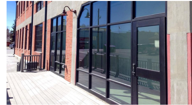
Commercial-grade windows and doors at business entrances in Rock Springs, WY. Windows and doors were retrofitted to complement the architecture of the historic building.
