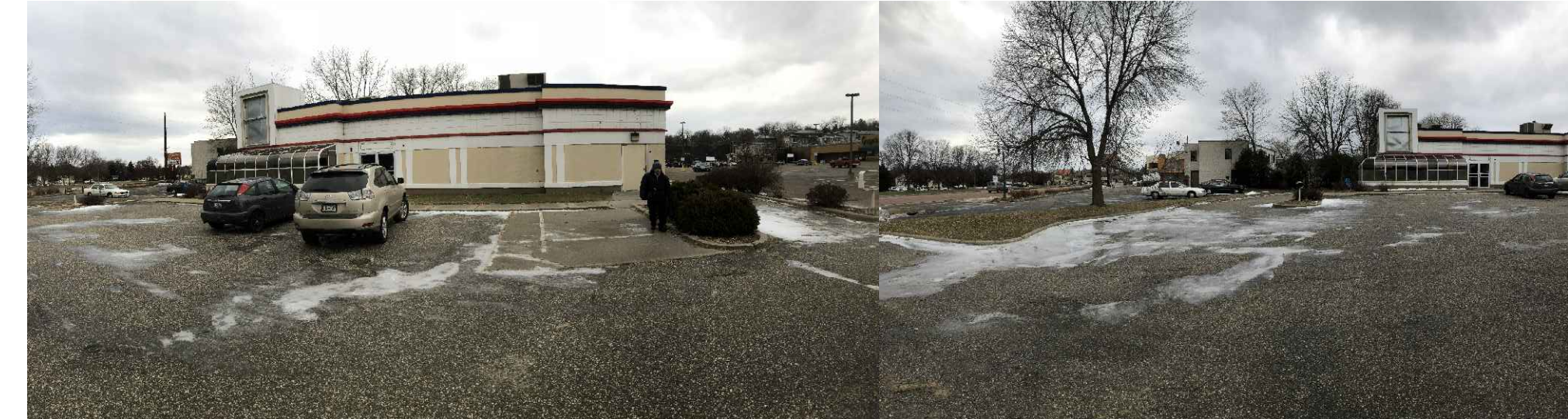
EXISTING CONDITIONS PHOTOS
