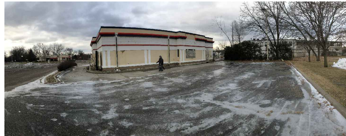
EXISTING CONDITIONS PHOTOS
