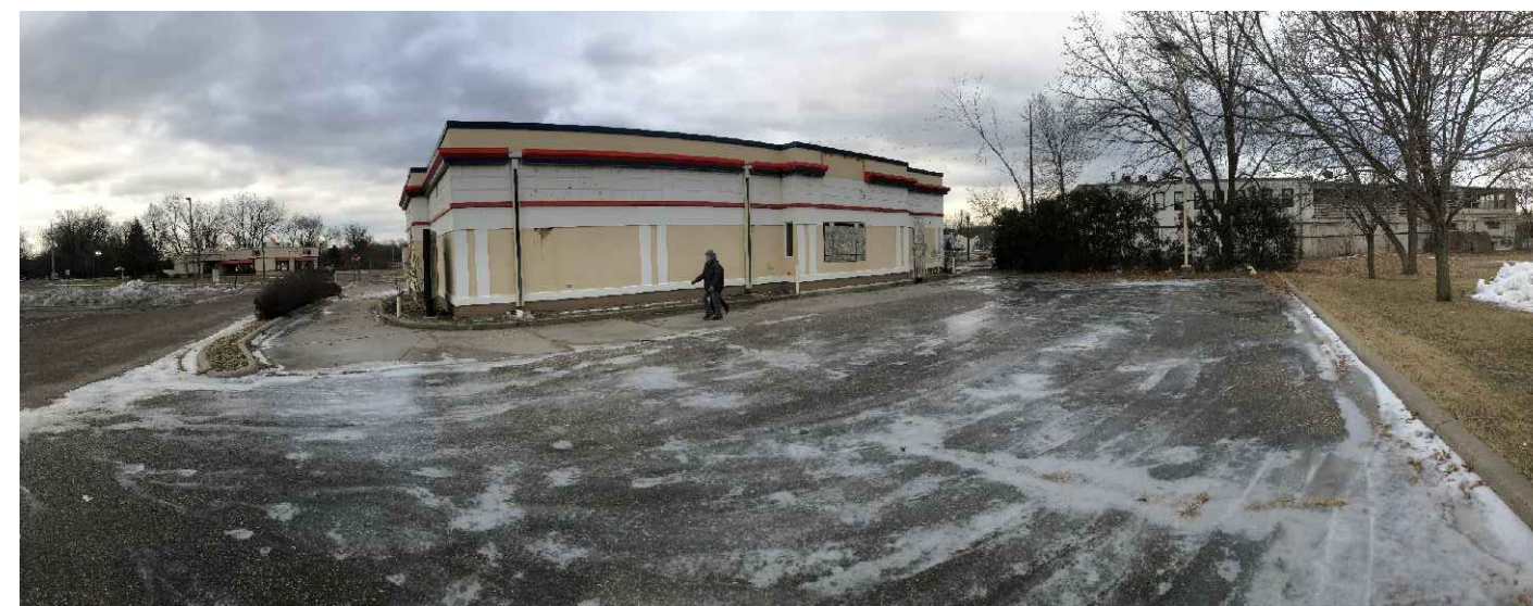
EXISTING CONDITIONS PHOTOS
