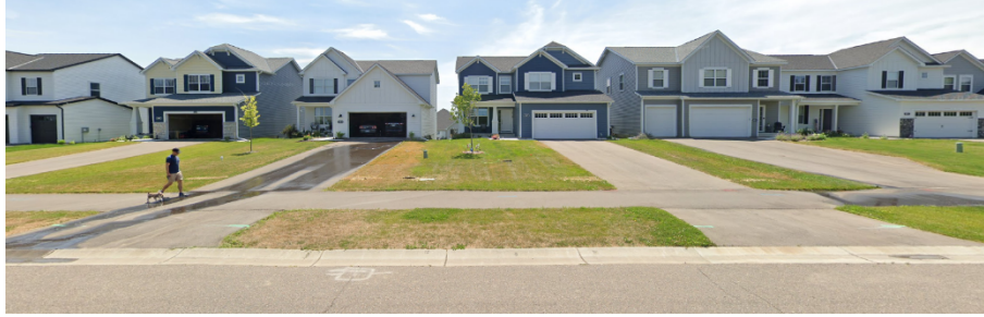
Figure 7: existing homes on the south side of Spring Creek Drive
