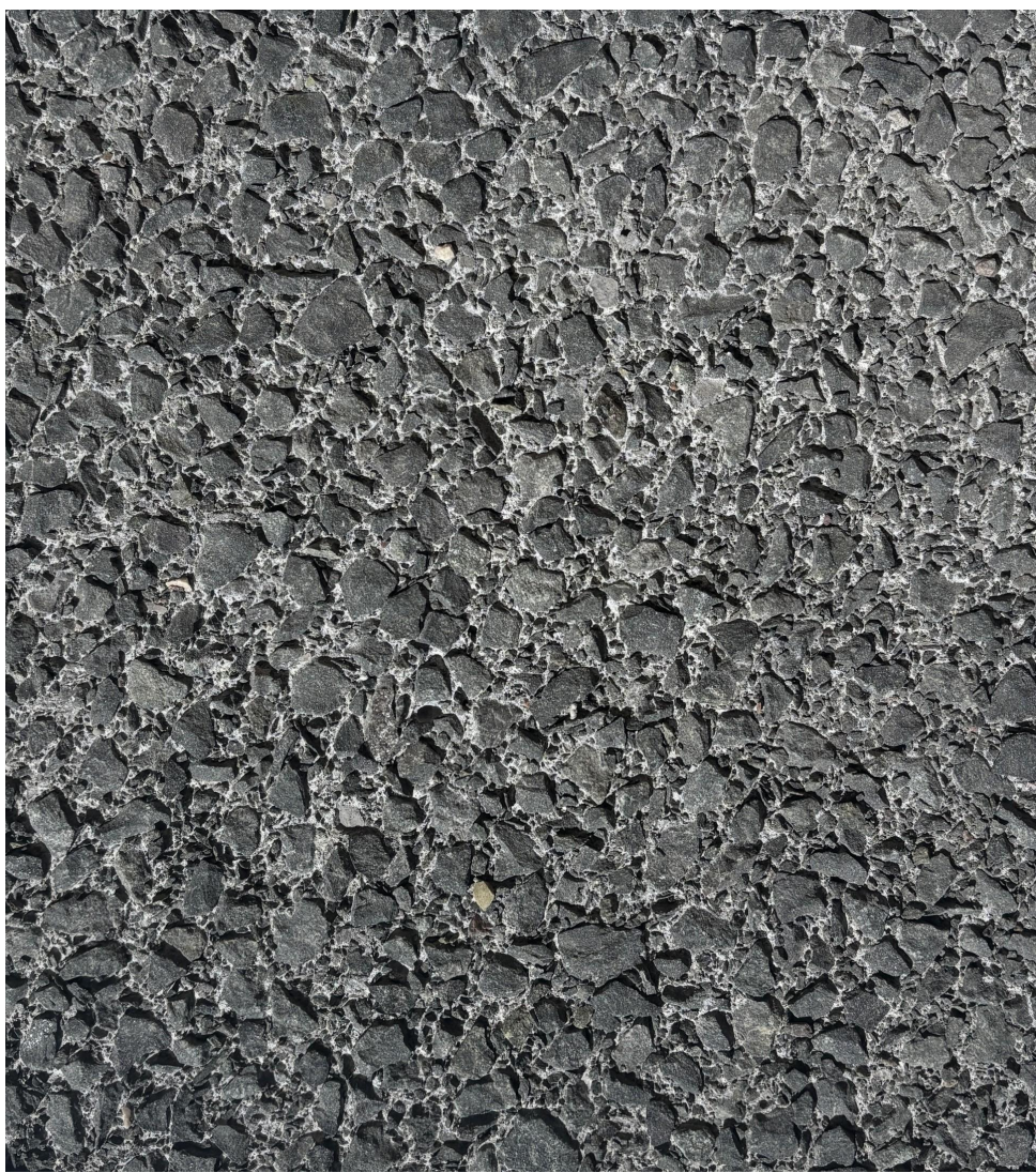
TOP SIDE EXPOSED AGGREGATE FINISH
