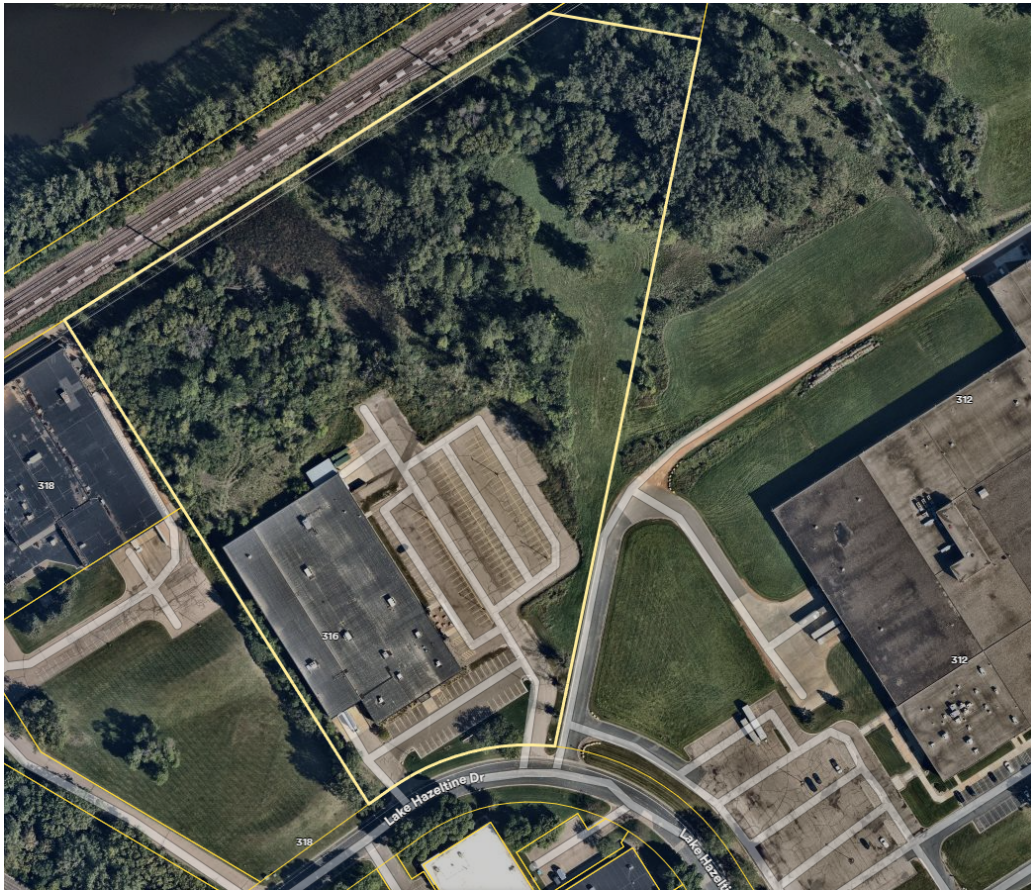
Figure 2: Extents of 316 Lake Hazeltine Drive site with existing Building 316 and greenfield space for the building addition.
