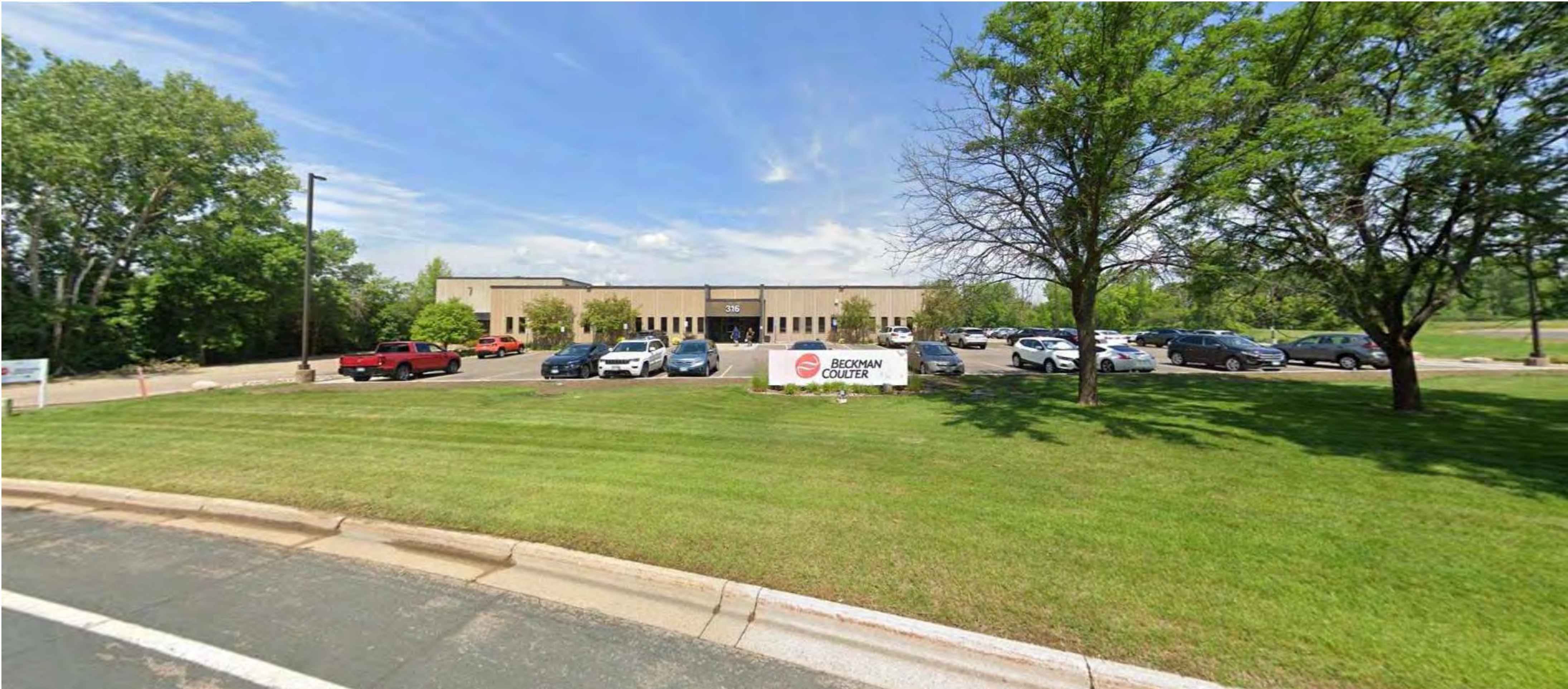
1. VIEW FROM LAKE HAZELTINE DRIVE, LOOKING NORTHWEST
