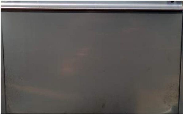
METAL PANEL CLADDING
