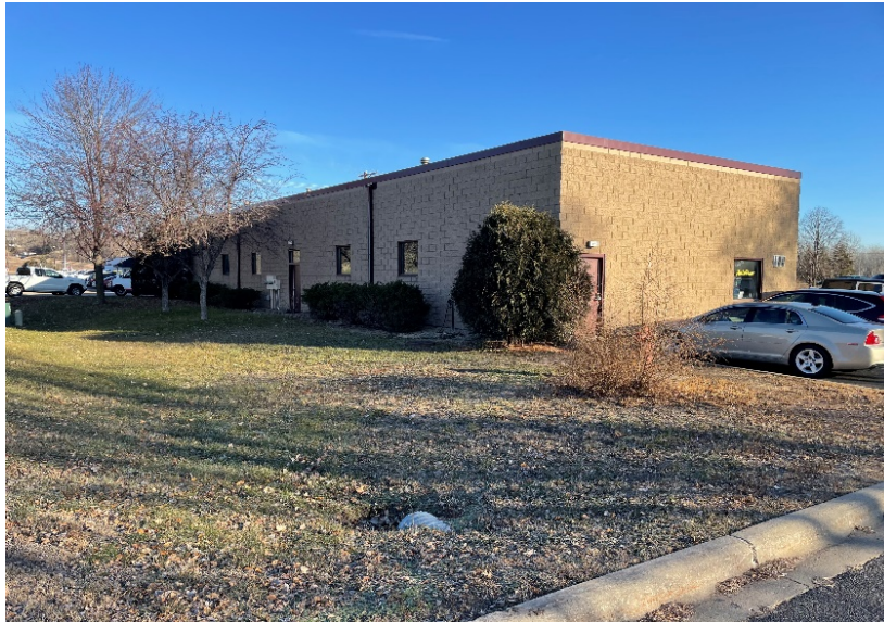
Figure 1: Existing Building viewed from southwest on Audubon
