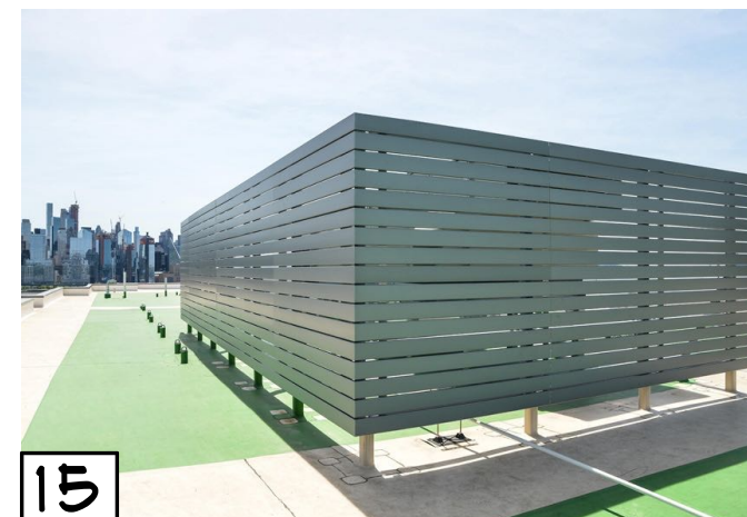
15 MECHANICAL SCREEN WALL PREFINISHED ALUMINUM SLATTED LOUVER
