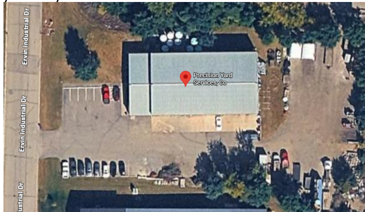
Figure 3: Existing PYS in Jordan
