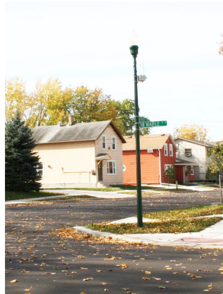
New Fiberglass Street Lighting
