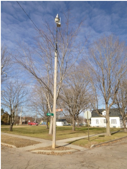
Existing Street Lighting
